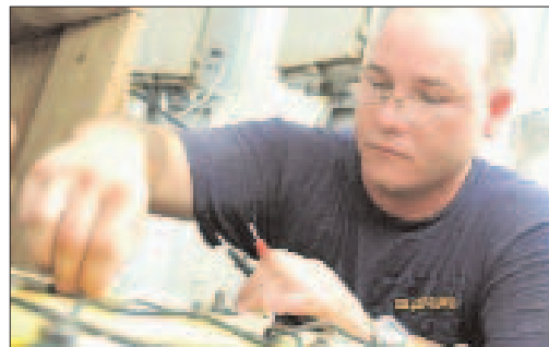
Seaman Apprentice William Mason tests the lighthouse's batteries.
